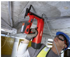
Threaded rod attachments to concrete
