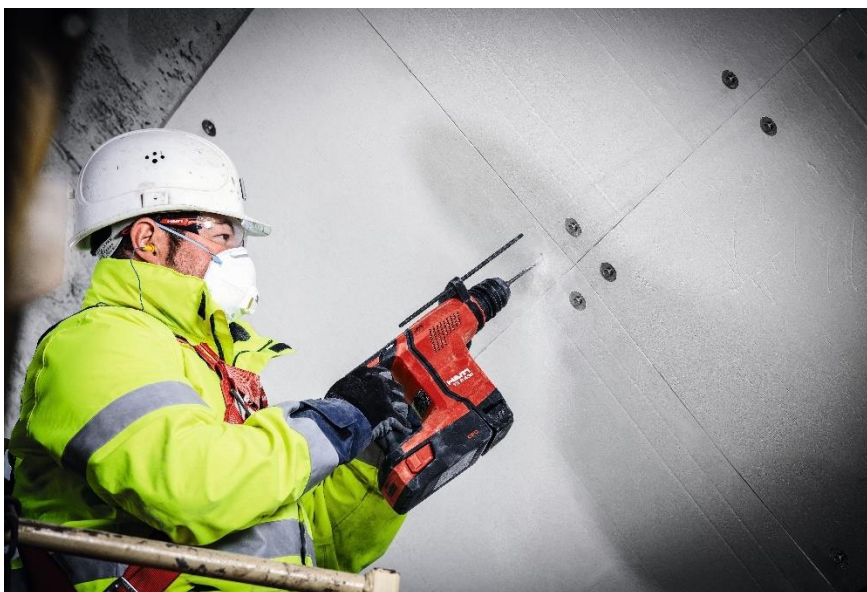
Fastening of pre-fabricated fire protection boards
