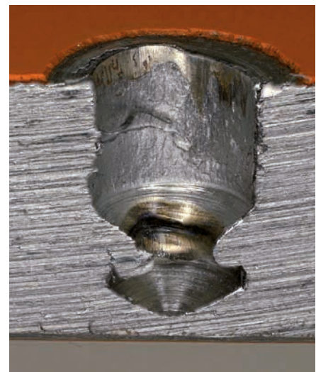
Steel base material after 10 years of exposure to sea water and pull-out of the X-BT fastener. The hole appears clean and no evidence of corrosion is visible.
