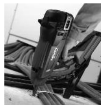
Conduits & pipes with metal or textile band
