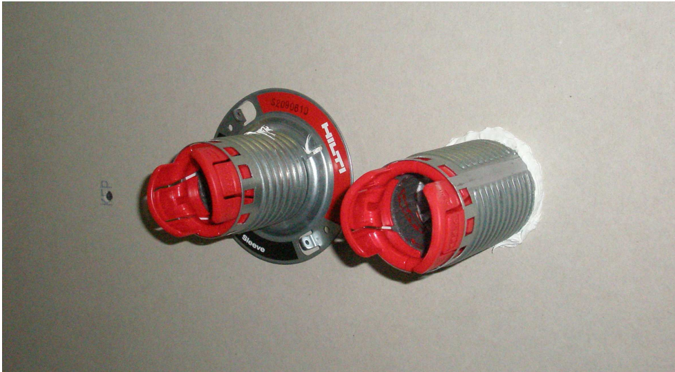
Fig. 2 Installation of cable penetration assemblies
