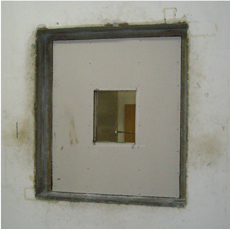
Fig 2 Photo of metal stud partition with penetration
